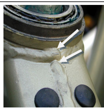
Arrows show where to file if necessary.
